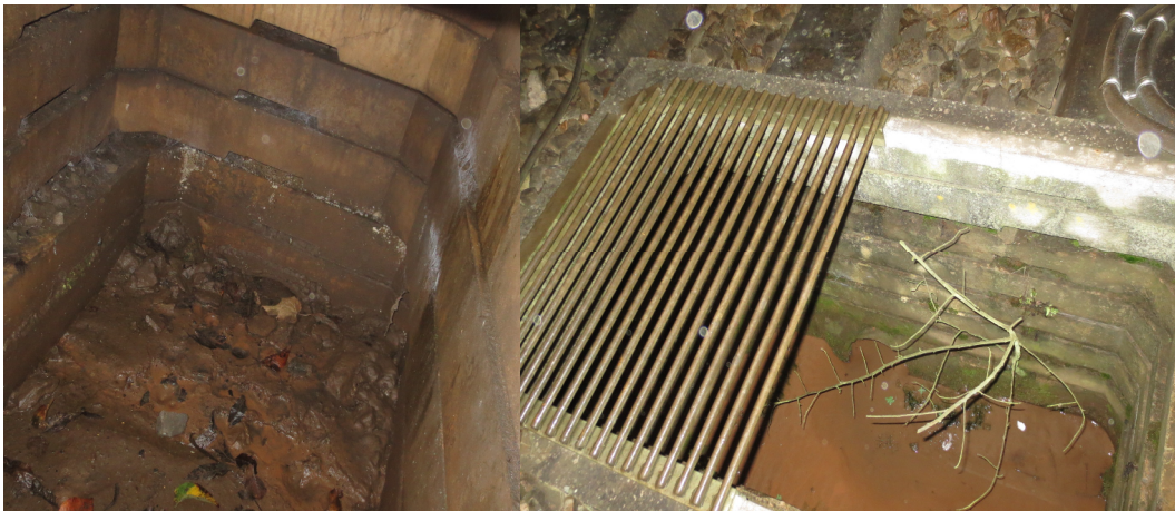
Figure 1: Indicative CAT1.1 catchpit condition
