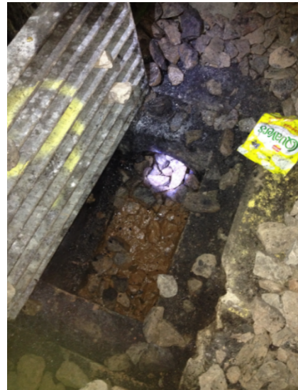
Figure 7: Informal chambers within Pill tunnel; observed as twin wall pipes with top half cut out with concrete frame and steel grate.
