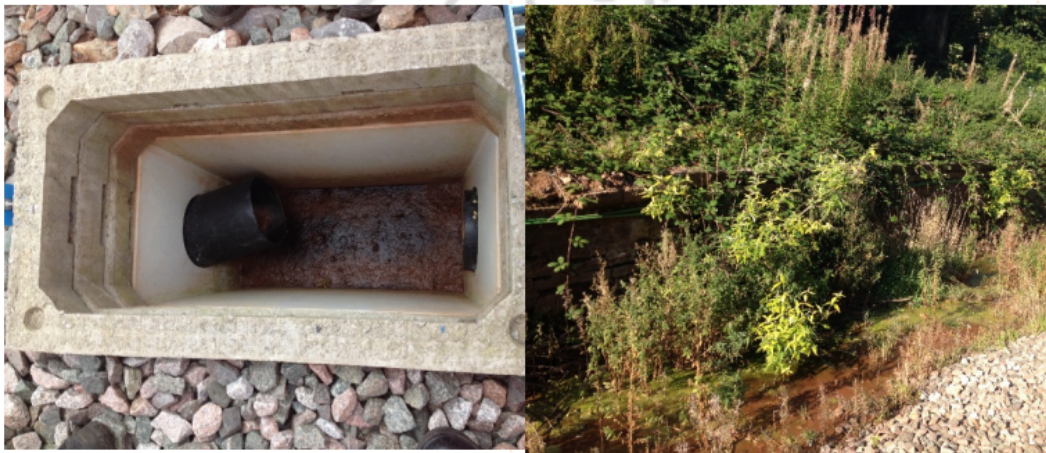
Figure 10: a) Final catchpit (condition indicative of all d/s catchpits) b) standing water observed within the cess
