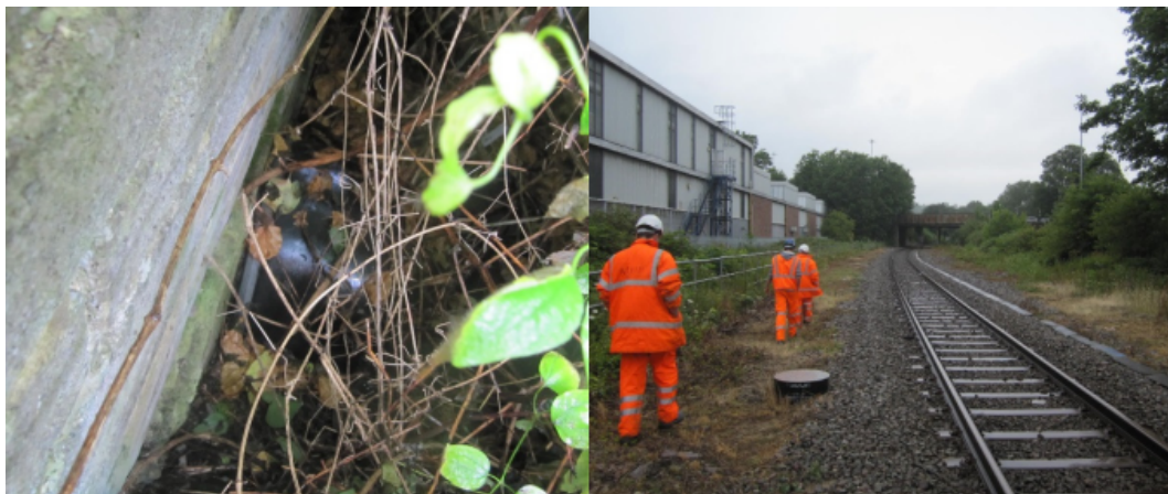
Figure 4: a) Outfall to concrete lined ditch, b) Route showing AQUA SE catchpits in the Dn cess (handrail to LHS of picture is on top of the outfall ditch). Note the lids have now been changed for grated steel lids.
