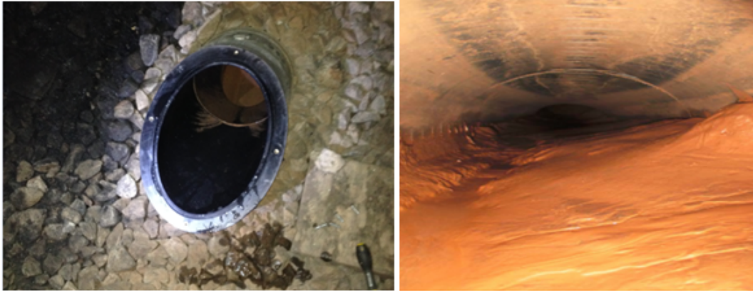
Figure 8: Rodding points in the Up cess showed extensive siltation within the system
