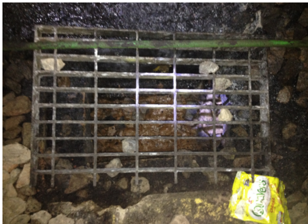
Figure 7: Informal chambers within Pill tunnel; observed as twin wall pipes with top half cut out with concrete frame and steel grate.
