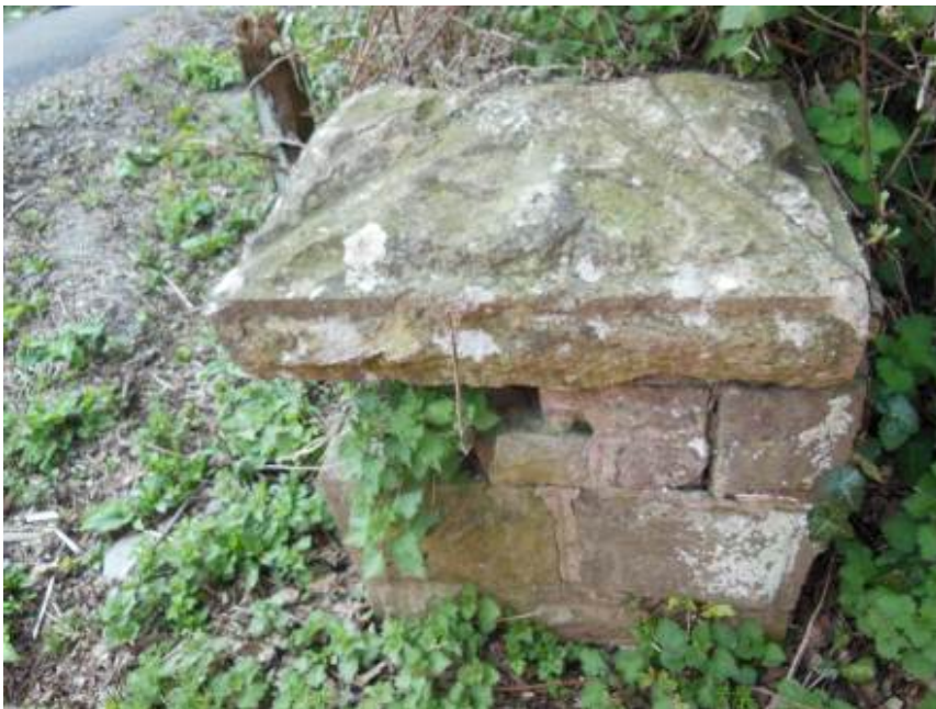
Figure 37 - Stones under newel cap missing
