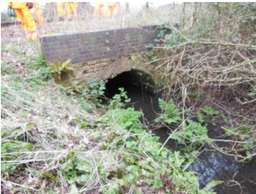
Figure 29 – Culvert B: view South side of line: spalled masonry and open joints visible
