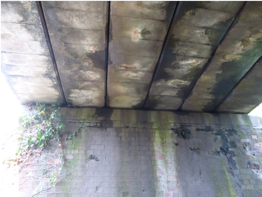
Figure 48 – Bridge soffit: isolated spalling and visible corrosion
