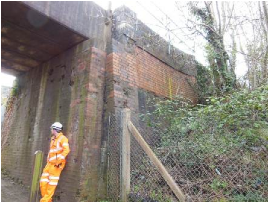
Figure 49 – Spalling to masonry on buttress and abutments
