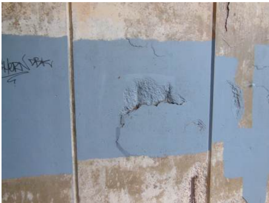
Figure 44 - Spalling to the abutments
