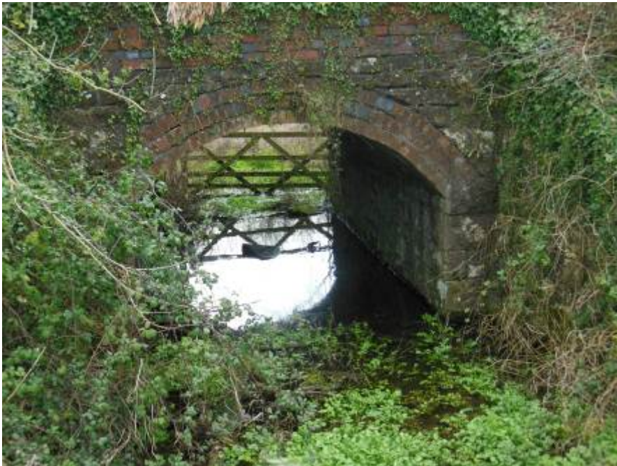
Figure 40 - Cattle creep: open joints visible in the arch rings and spandrel wall
