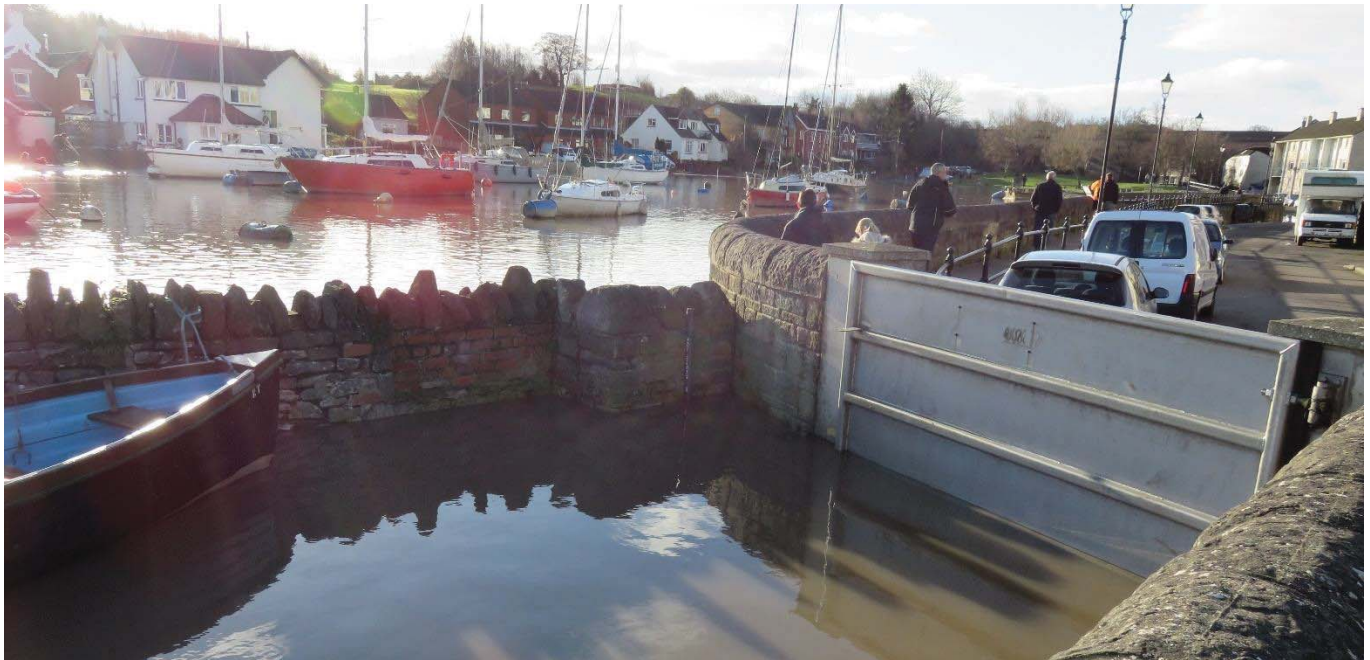
Figure 25: Existing flood defences in operation at Pill
