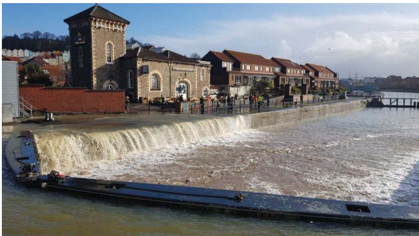
Figure 37: Overtopping at Junction Lock during March 2020 tidal surge
